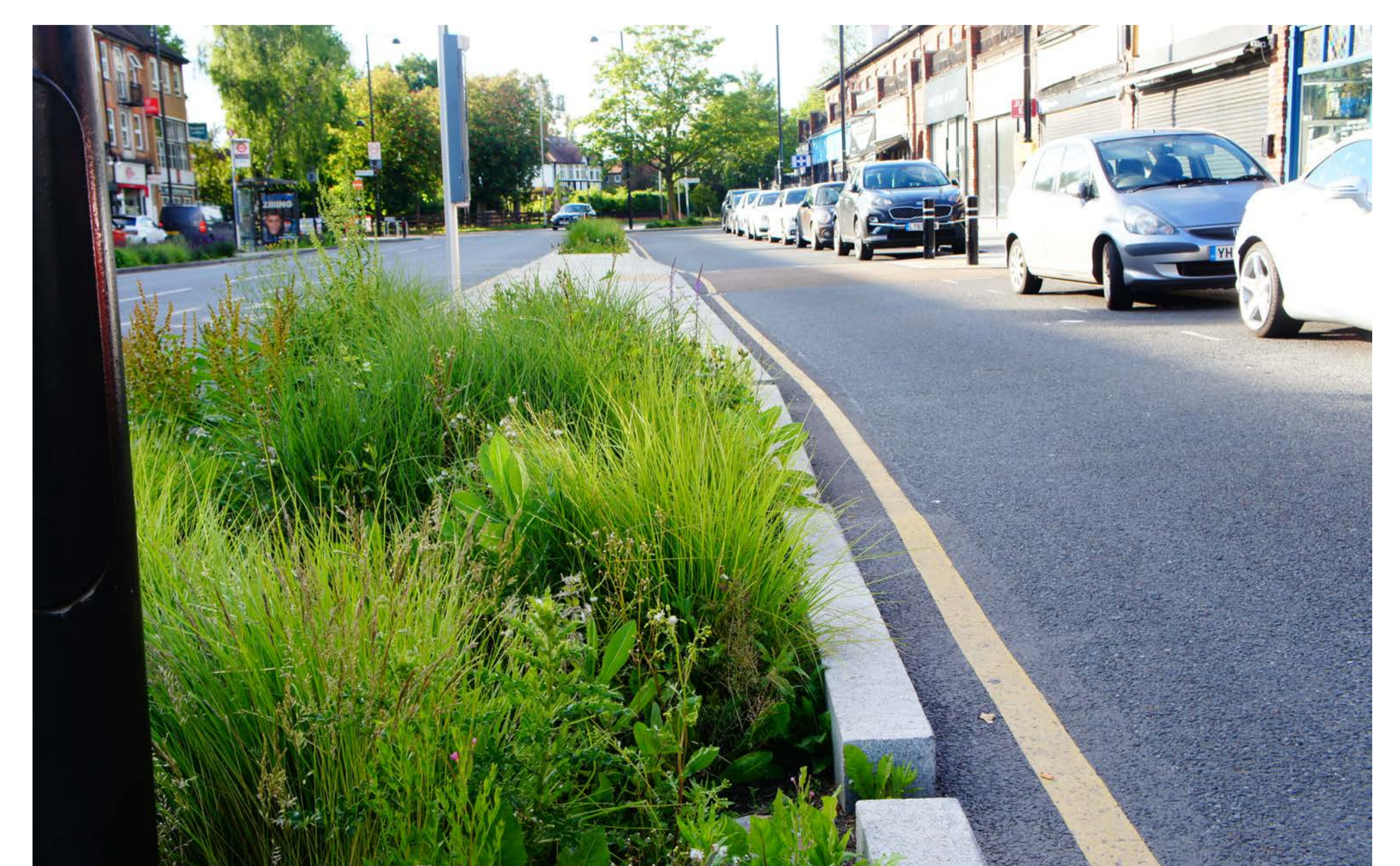
Typical rain garden and edging
