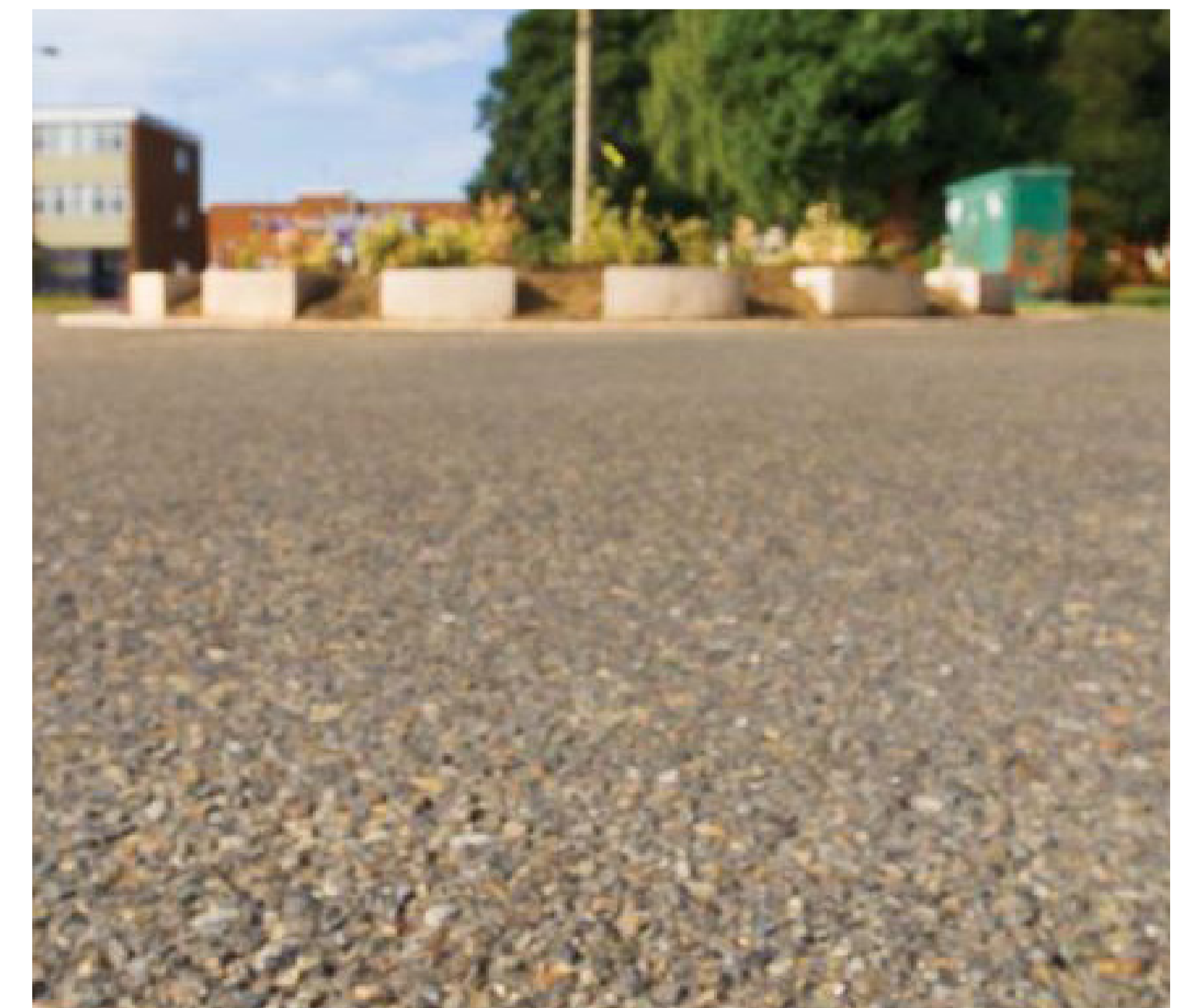
Porous asphalt with garden bed
