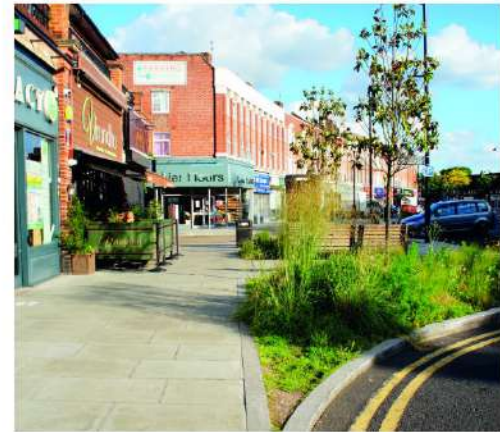
Typical rain garden planting for SuDS
