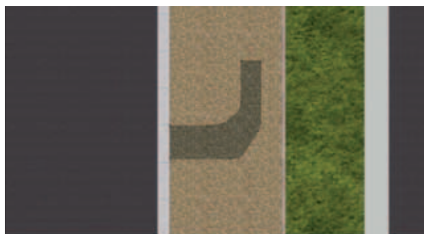
Poor reinstatement following excavation of path
