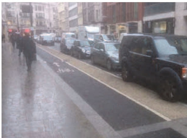
Contraflow cycle lane protected by parked cars and door zone, Hanover Street, LB Westminster
