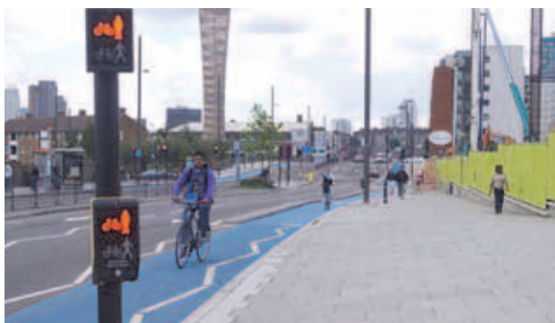
Segregated track, with protective island, CS2 Stratford
