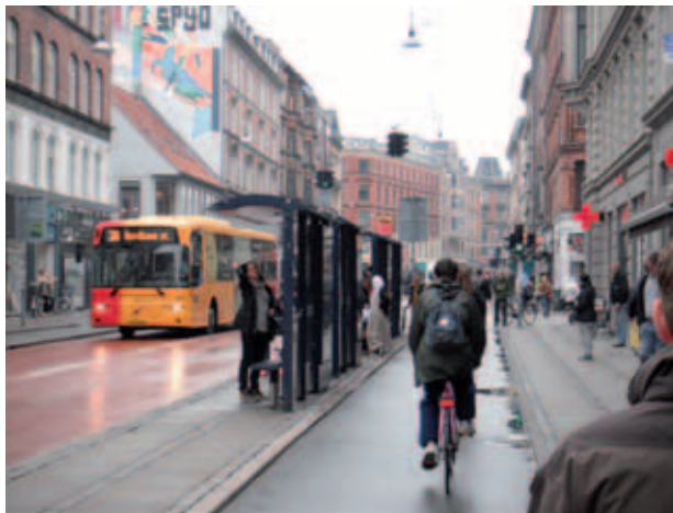
Stepped cycle track with bus island in Copenhagen, Denmark
