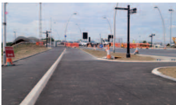
Splay kerb on segregated track, Ruckholt Road
