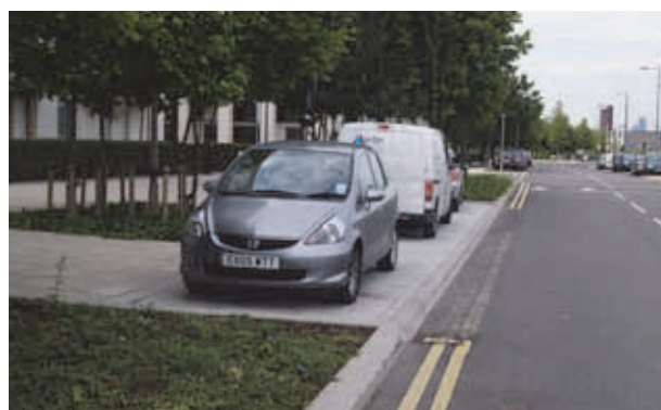
Inset car parking with door zone, Queen Elizabeth Olympic Park
