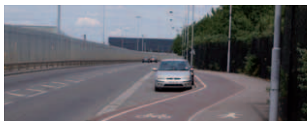
Existing inset parking bay with segregated cycle track, Orient Way
