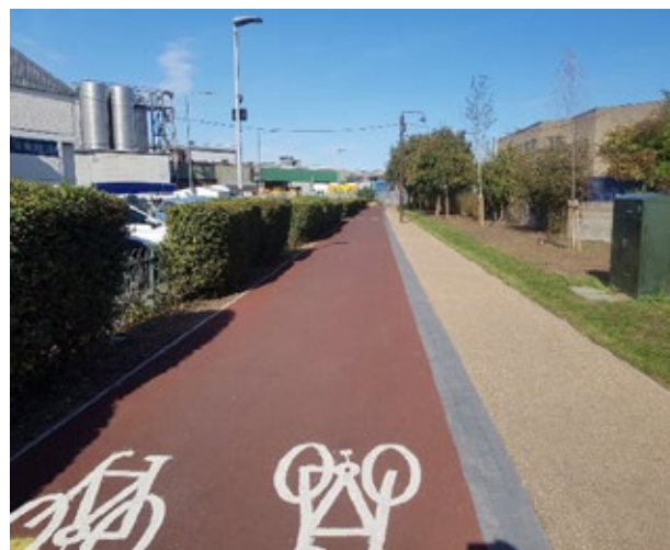
Segregated cycle track on the Black Path, Argall Estate
