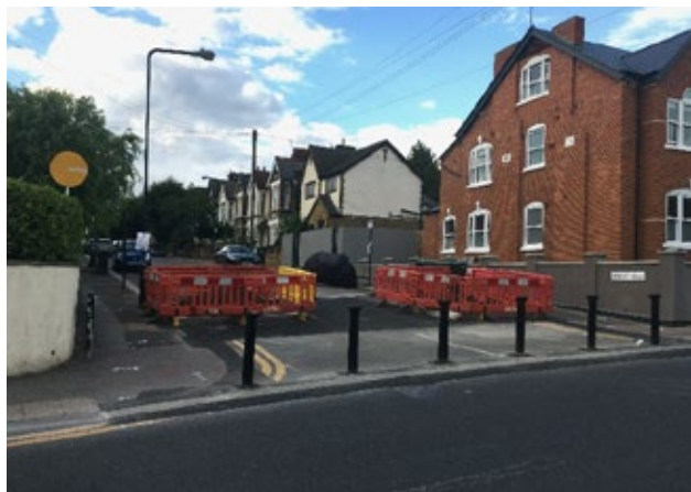
Construction on Seaford Road modal filter
