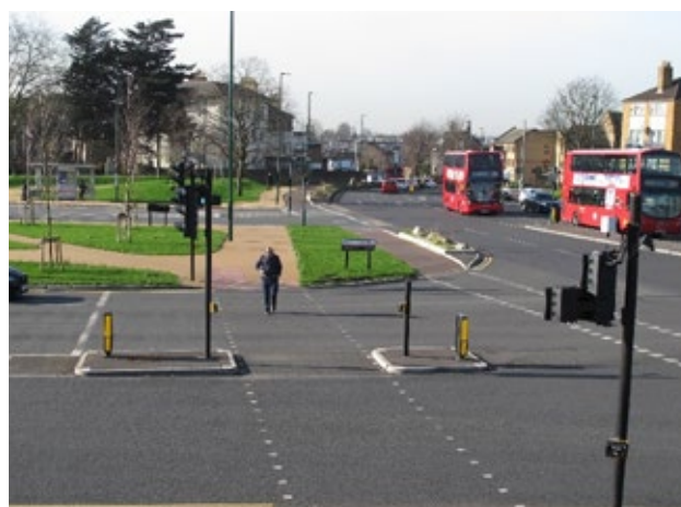
Completed Whipps Cross transformation
