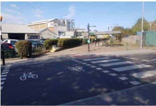
Shared cycle and pedestrian crossing on Argall Way
