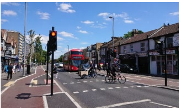
Completed flagship scheme - Lea Bridge Road
