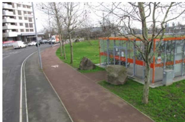
Segregated cycle track on Argall Way
