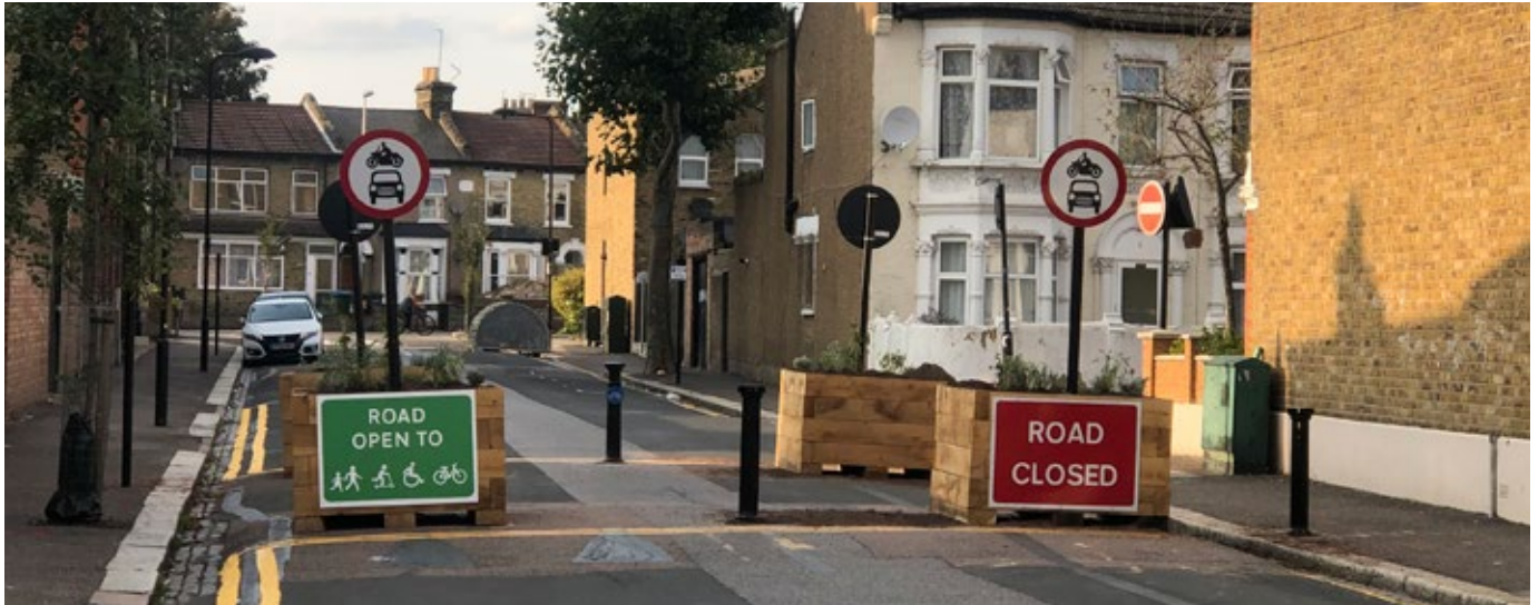
Image of existing modal filter on Blenheim Road
