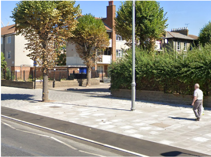
Existing continuous footway at the Hoe Street/ Grosvenor Park Road junction
