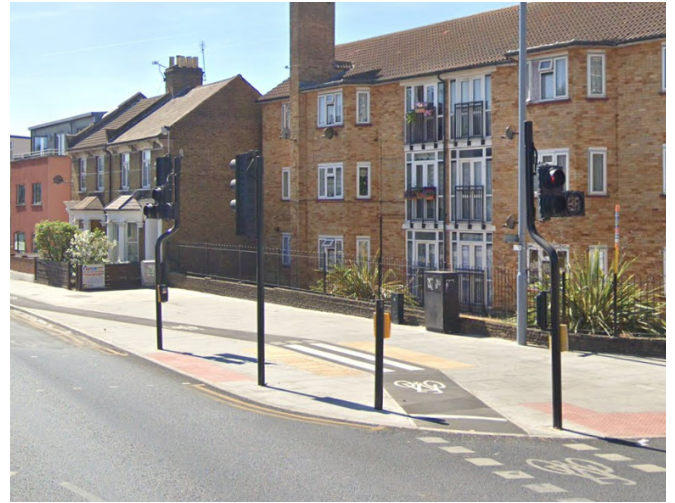
Existing separated cycle track with pedestrian crossing at the Orford Road/ Queens Road junction
