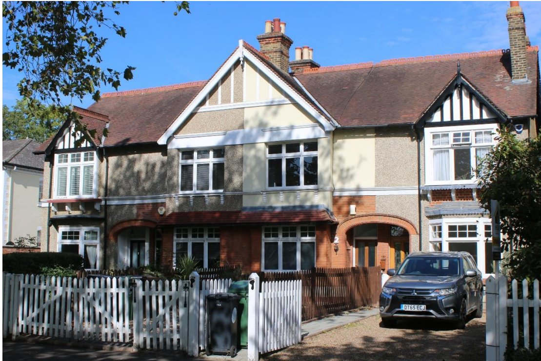
SMOOTH RENDER AT THE FIRST FLOOR OF NO.2 JUBILEE VILLAS DISRUPTS THE OVERALL LOOK OF THE ENTIRE TERRACE, WHICH ORIGINALLY WOULD HAVE BEEN ENTIRELY ROUGHCAST RENDER.
