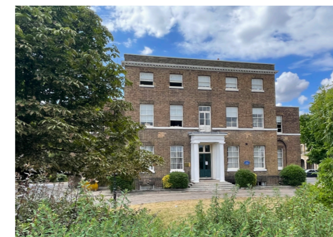
Leytonstone House (built approx 1800)
