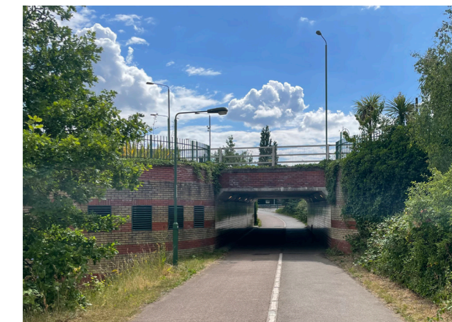
Pedestrian and cycle path under Green Man roundabout
