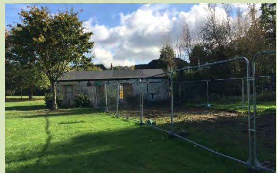
Building at Highams Park is being refurbished.
