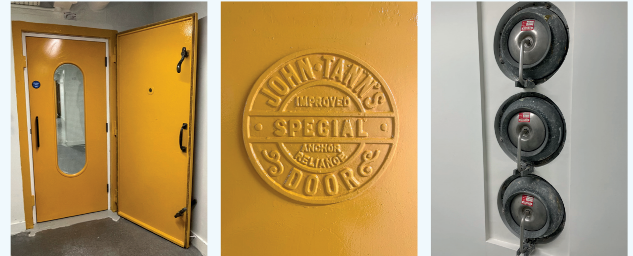
Below: The Town Hall basement which retains its steel airtight doors.
