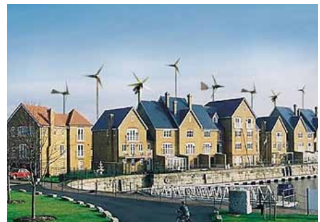
Renewable energy features which are not discreet may have a detrimental impact on the street scene
