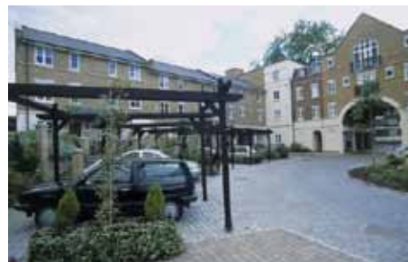
Parking designed as an integral part of the street scene and not as an after thought
