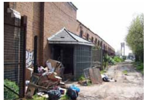
A pedestrian route along the back of one of the Borough's housing estates which is used for dumping rubbish
