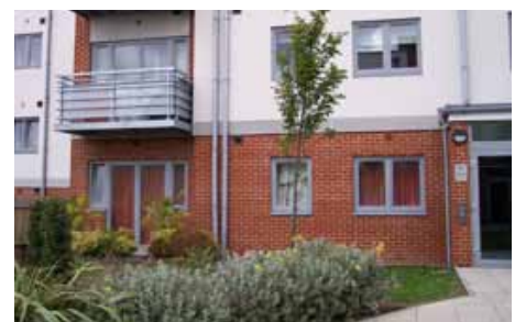
Bedrooms on the ground floor often have permanently closed curtains
