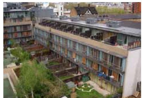
Private and communal spaces need to be usable and of high quality (Transition Culture)
