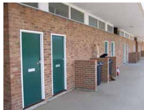
A housing development with no windows and inactive frontages
