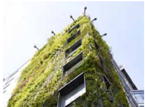
Living walls reduce heat loss and contribute to biodiversity (Kayak)
