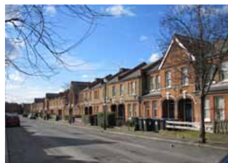
Typical two storey development in Walthamstow
