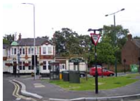
Poorly sited utilities
