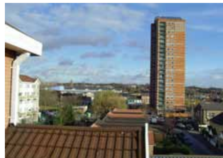
One of the few remaining 1960s tower blocks in Waltham Forest
