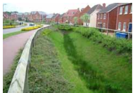
Sustainable urban drainage system (SUDS) (Cyria)
