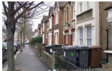
Consideration needs to be given to the storage of wheelie bins as part of overall design
