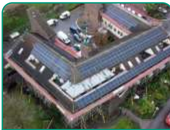
Longfield House sheltered accommodation Solar panels
