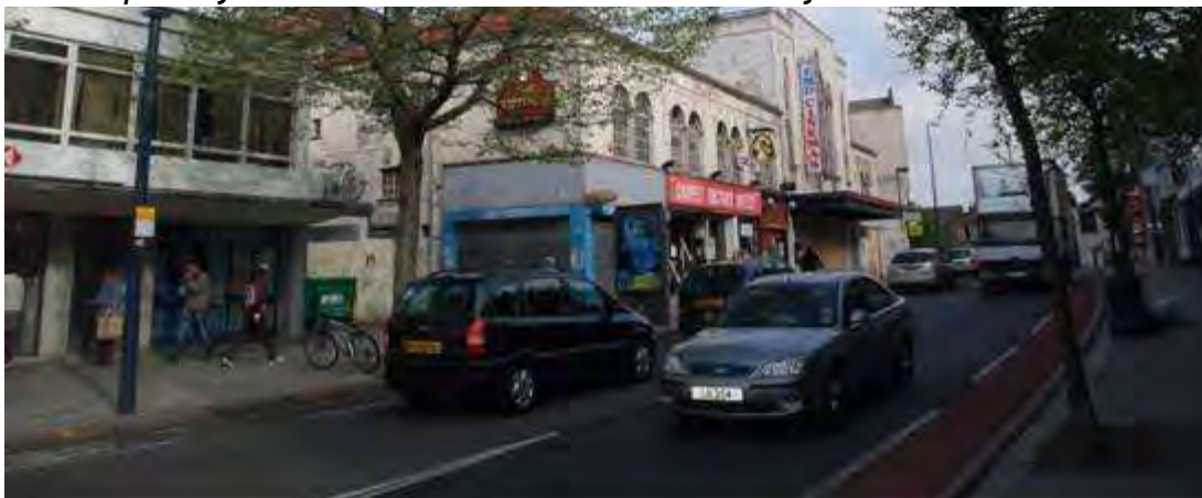
Figure 10: The side wing of the cinema provides the opportunity to create a discrete entrance with a strong street presence. A void space behind provides the opportunity to provide access to screens at a higher level and also possibly to create additional screens over the lobby area.
