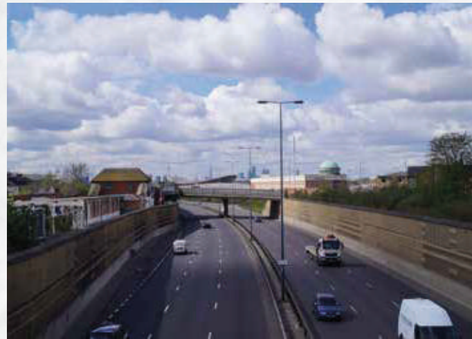
View from Langthorne Road bridge
