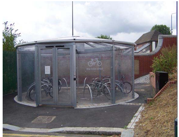
Secure bike shed with smartcard entry system at Leyton station
